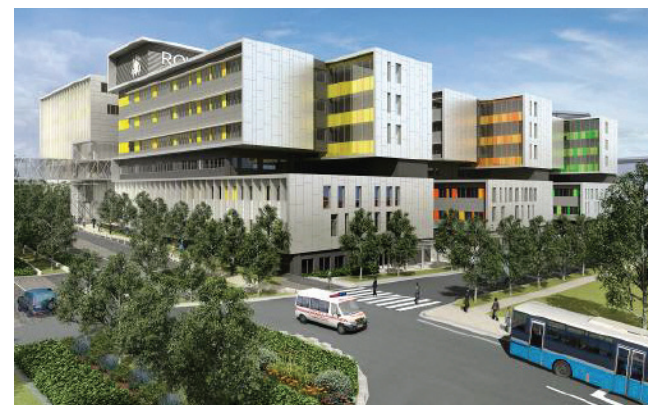
ROYAL NORTH SHORE HOSPITAL NEW BUILDING
