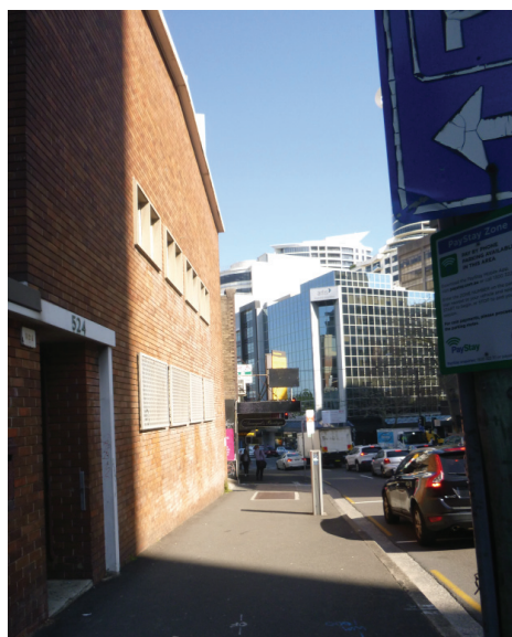
NARROW FOOTPATH ALONG TELSTRA EXCHANGE FACADE
