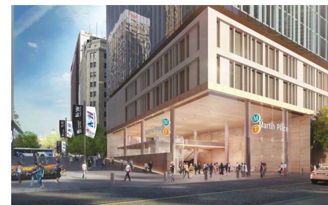
MARTIN PLACE STATION
