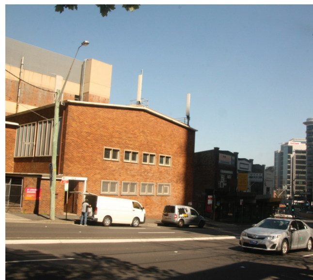
TELSTRA EXCHANGE STREET FRONTAGE TO PACIFIC HIGHWAY
